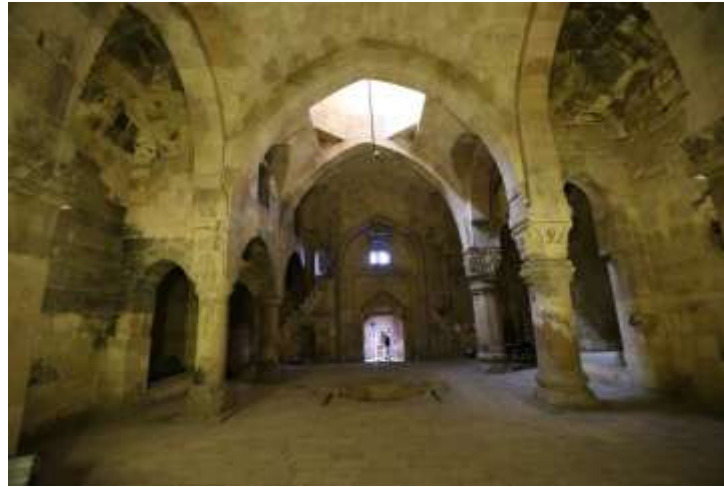
Figure 8. Inside the hospital, looking to the west
