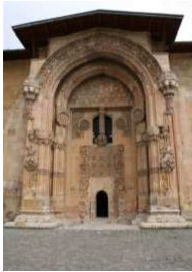
Figure 6. The main door of the hospital
